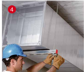
4 Mechanical & electrical, HVAC
